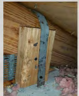
Correct strap with blocking
