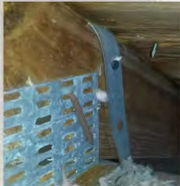
Single wrap front side with 2 nails
