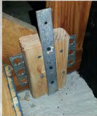
Strap that had spacing issues we corrected by blocking
