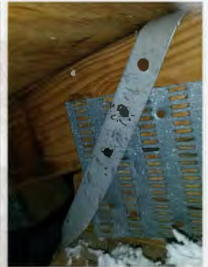
Wrap with minimum 2 nails on front 1 on backside
