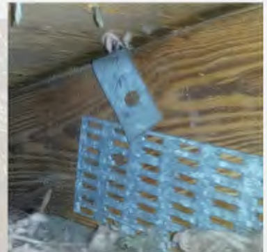
Single strap back side with one nail
